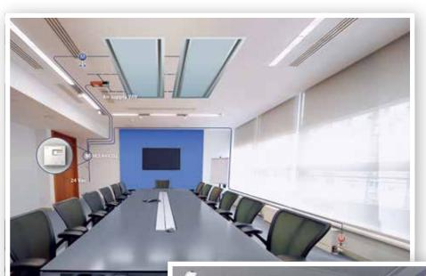
In conference rooms, HLS 44–CO2 (page 28) can control chilled beams with cooling and a damper actuator for ventilation if the CO<sub>2</sub> values are too high, or if cooling is required. Heating is controlled with radiators.
